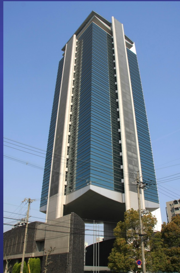
Unstable Looking Structure
